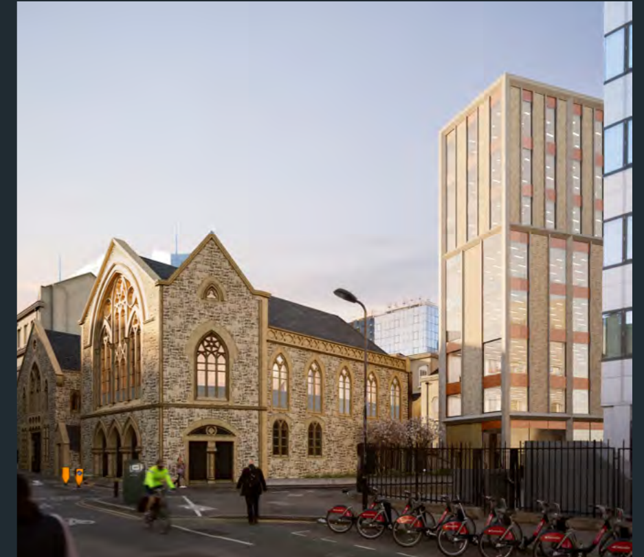
View from the South East along Leonard Street
